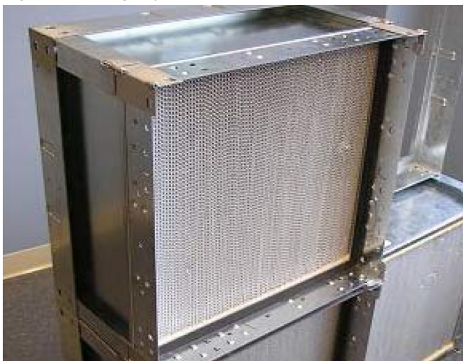
Figure 122: Properly Installed HEPA Filter
