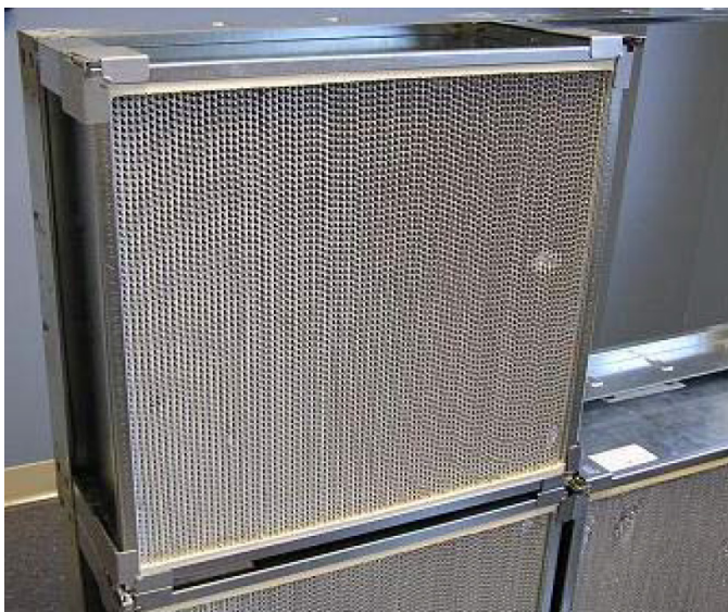
Figure 117: Properly Installed Filter Inside of the Frame
