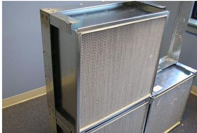
Figure 113: Filter Placed Inside of Frame
